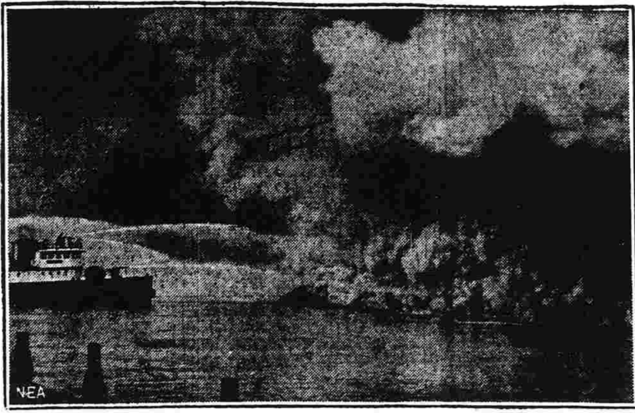
Behind these rolling clouds of smoke, raging flames were sweeping a $2,500,000 pier of the Cunard Line in New York when the picture was taken. More than 700 firemen, fifty pieces of land fire apparatus and a half-dozen fireboats fought to prevent the blaze from spreading to adjoining piers, and surgeons treated scores of persons affected by the smoke. The liner California was moved out into the Hudson river to escape the flames.
